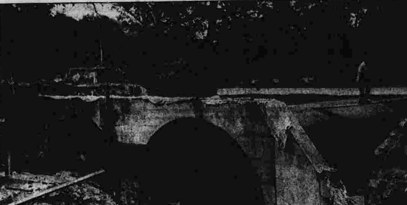
These two large culverts will replace the old bridge.
